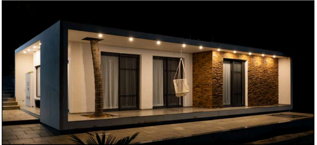
Natural stone rubble claddings to give rustic and raw finish.
